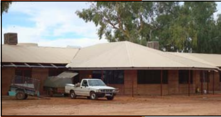
Boys dorm under construction
